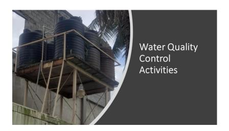
1.Each water tank should be cleaned and sanitized QUARTERLY to prevent micro-biological accumulation and potential contamination.
